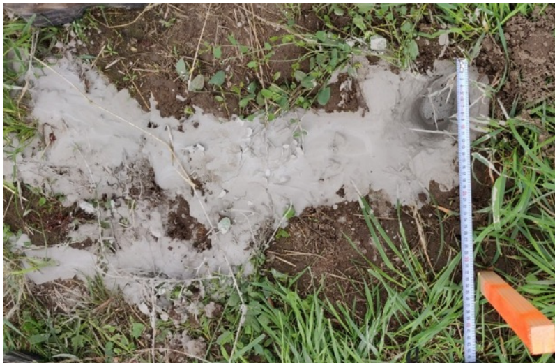
Figure 14 Entry point filled with fast-setting concrete
