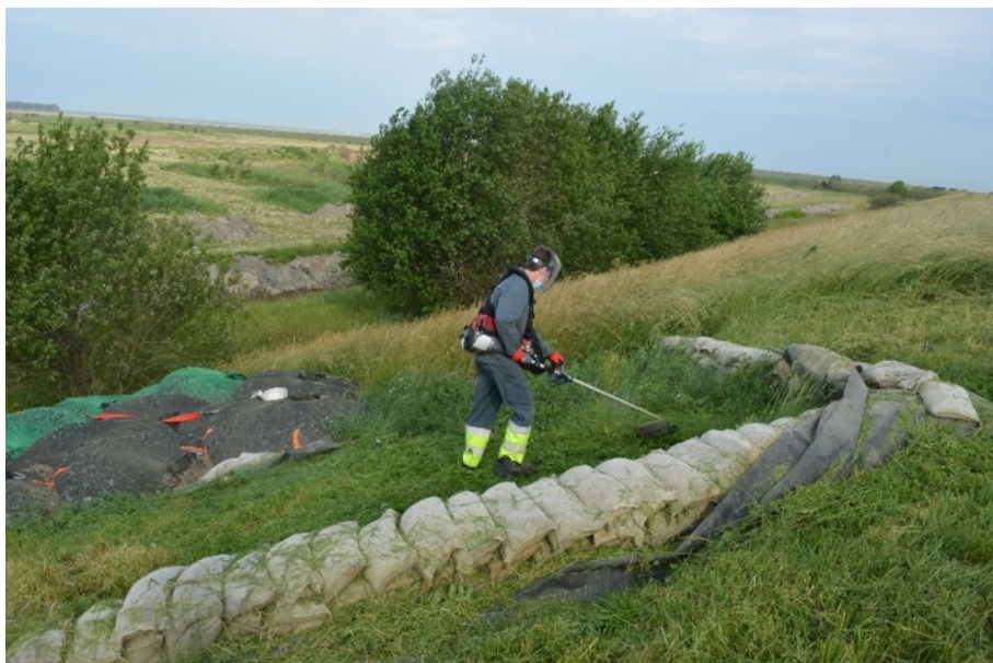
Figure 8 Preparation of test location, mowing grass
