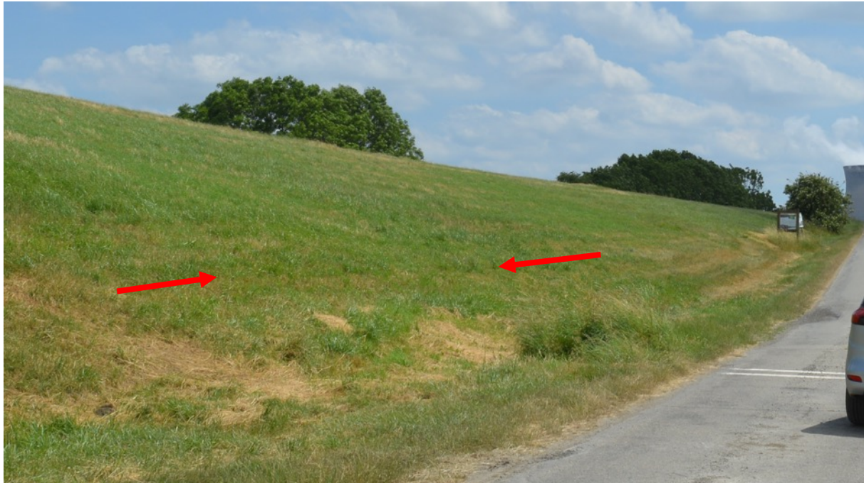
Figure 4 Rip observed at Dutch location 2 meters above a small reed vegetation, shown in both pictures.
